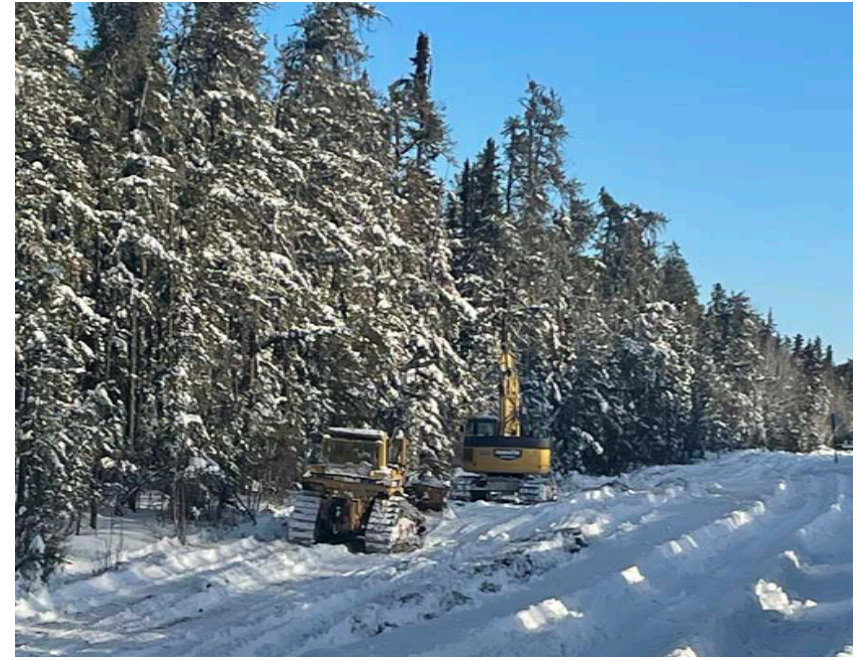
Equipment clears the ditches ahead of the installation of fibre cable along Highway 106.
